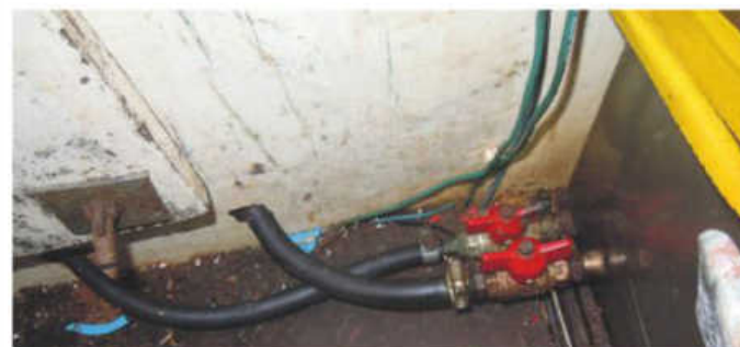
The bottom of the tank, showing the supply from tank to engine sited above the sump outlet that feeds into the polishing loop
