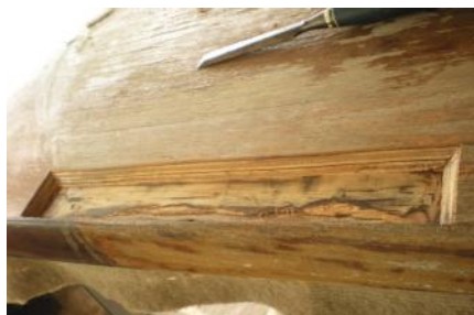
Trimmed back to sound wood ready for a new piece of ply to be scarfed in
